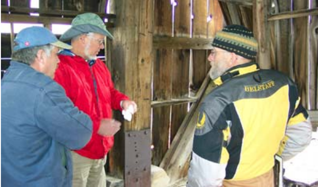
MARK YOUNG, BOB RISCH AND CHRIS GEORGE DISCUSS STABILIZATION INSIDE THE YANKEE GIRL HEADFRAME BUILDING.
